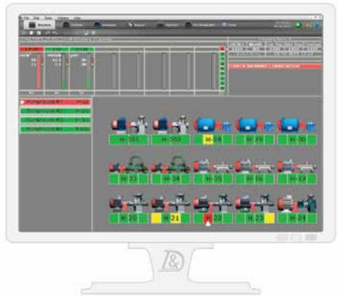
Figure 3. The Monitor mode of the COMPACS system – all machinery at a glance
